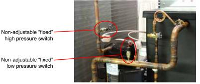
Typical placement of non-adjustable "fixed" pressure switches.
